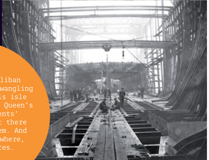
HOYFM.HW.H1074 Men working on internal construction of Iroquois Robert John Welch, (1859-1936); Harland and Wolff © National Museum NI, Ulster Transport Museum Collection
