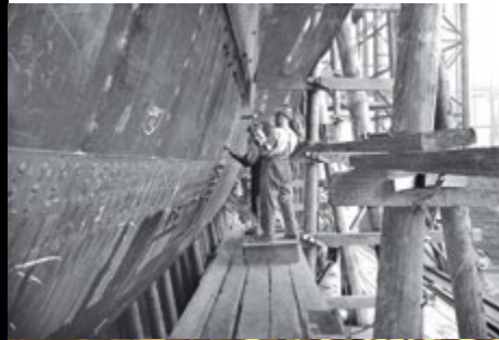
HOYFM.HW.H1915 Hand-riveters at work on Britannic Robert John Welch, (1859-1936); Harland and Wolff © National Museum NI, Ulster Transport Museum Collection
